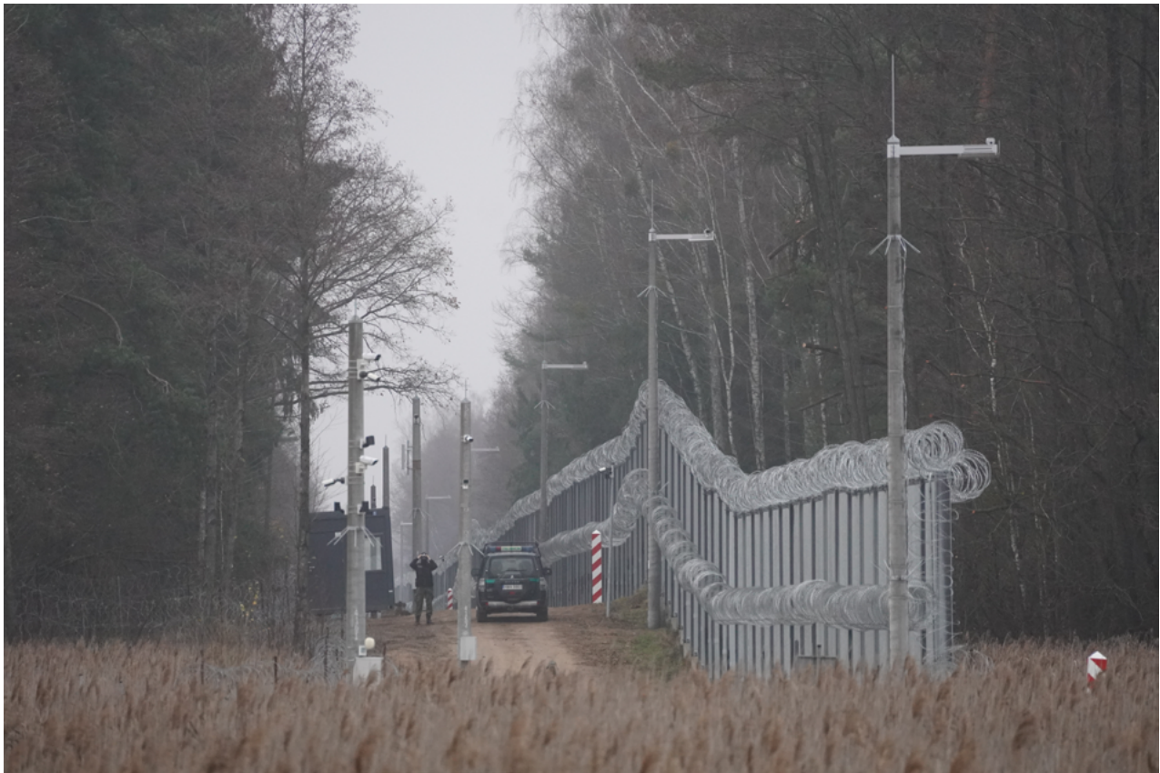
Figure 10. Border infrastructure at the Poland–Belarus border. The 5.5-metre steel fence and electronic surveillance system sit alongside older, low-tech methods of control, such as a patrol road and a guard scanning the treeline with binoculars. Photograph by Peter Teunissen, November 2024.
