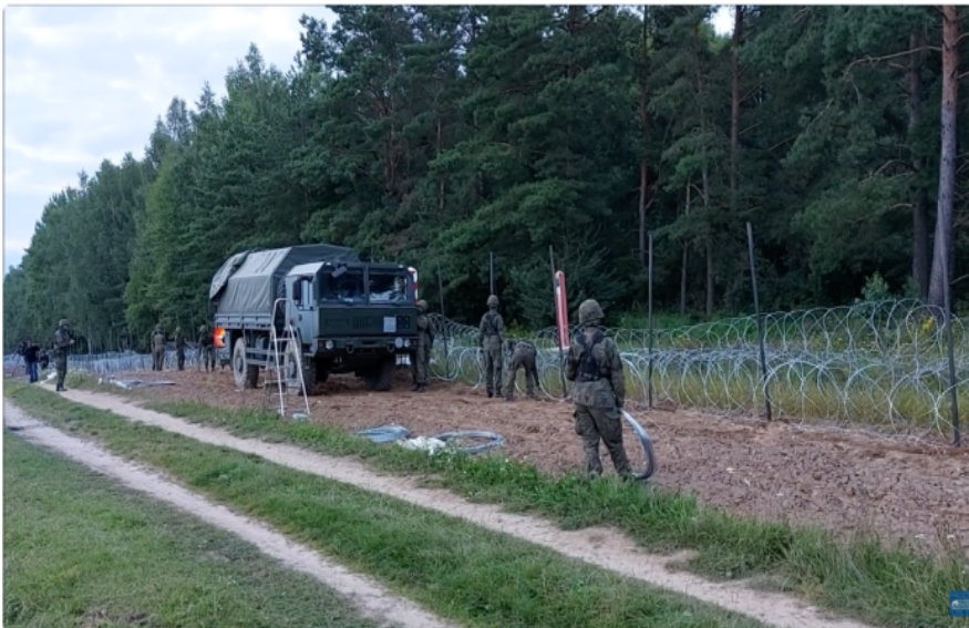
Figure 2.42. Polish soldiers install a concertina razor-wire barrier along the border with Belarus. Before this fence went up, the border in this heavily forested area was marked only by a cleared strip of land, also seen in the image, that was patrolled but with limited physical barrier. Screenshot from a video by Radio Białystok. 109
