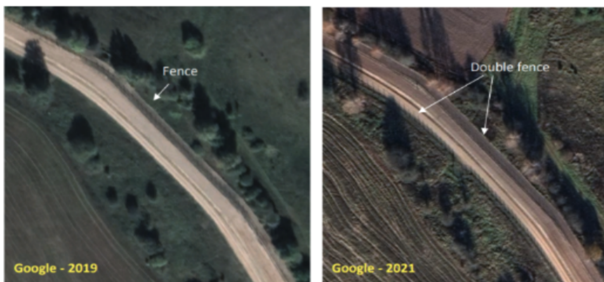
Figure 2.38. Satellite imagery analysis shows an additional metal fence in certain sections of the Belarusian border infrastructure. Its alignment is irregular: in some locations it extends deeper into Belarusian territory. Satellite imagery: Google Earth, Maxar Technologies, ©2019/2021.
