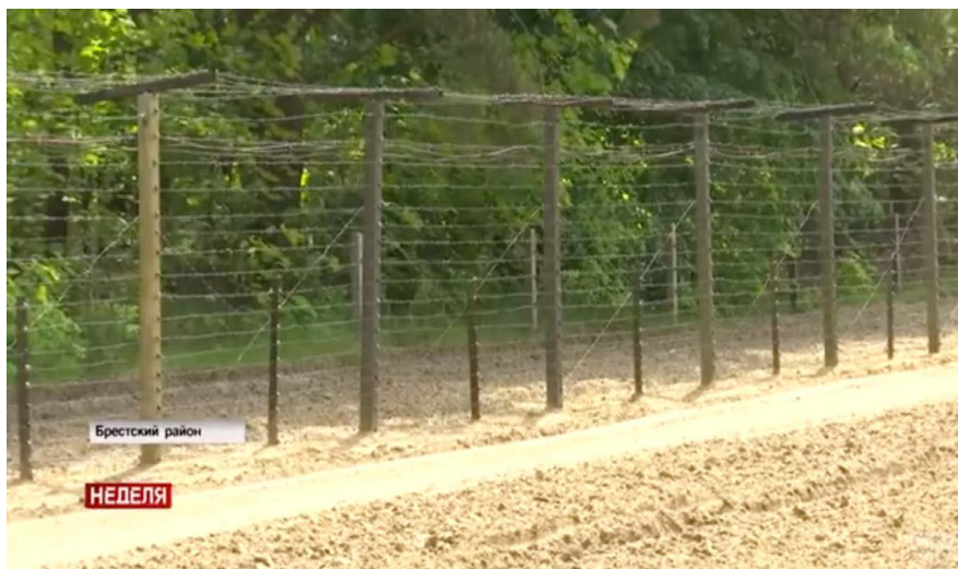
Figure 2.37. KS-100 system with a control strip of ploughed sand, Terebun Border Guard station, Belarus. Screenshot from a video by Pograneц.by, 2021. 196
