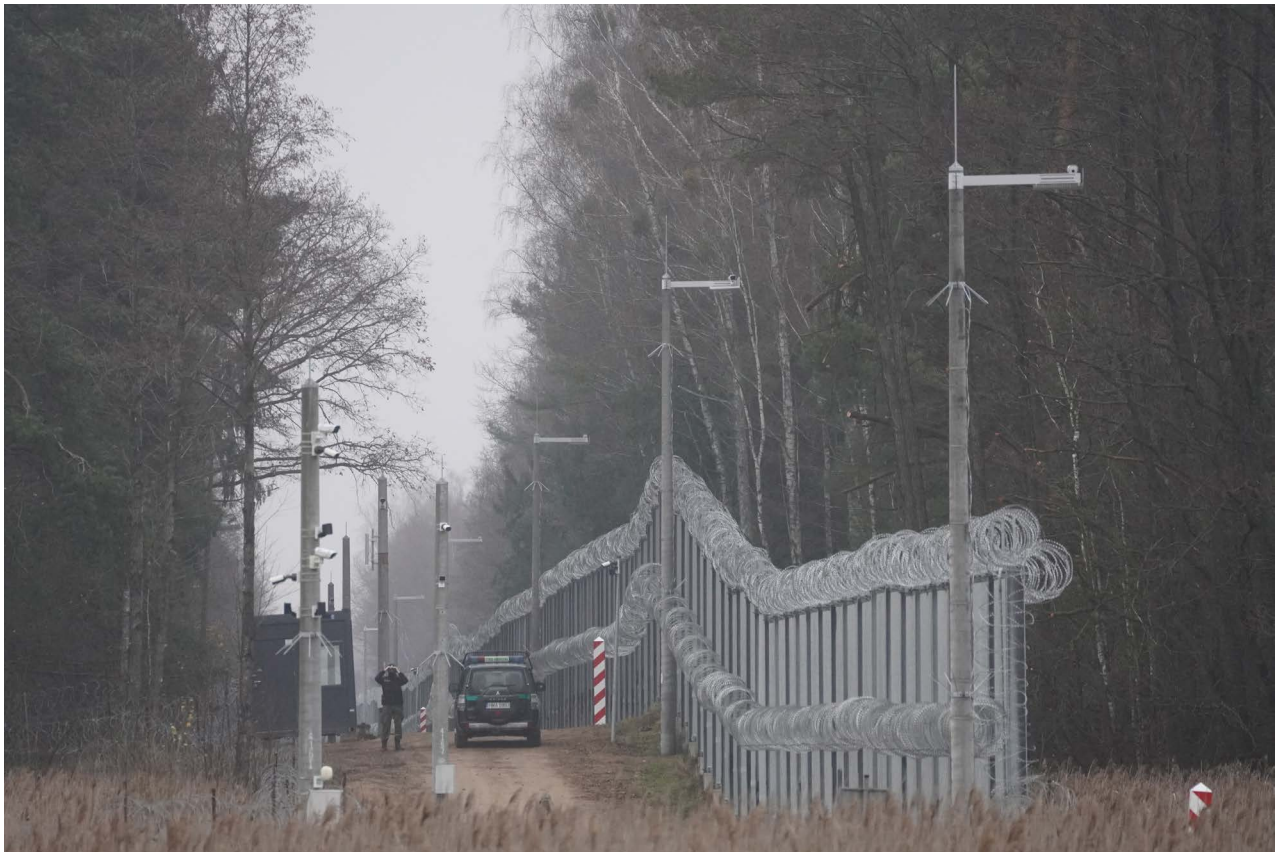
Figure 2.1. Border infrastructure at the Poland–Belarusian border. A 5.5-metre steel fence and electronic surveillance system sit alongside older, low-tech methods of control, such as a patrol road and a guard scanning the treeline with binoculars. Photograph by Peter Teunissen, November 2024.
