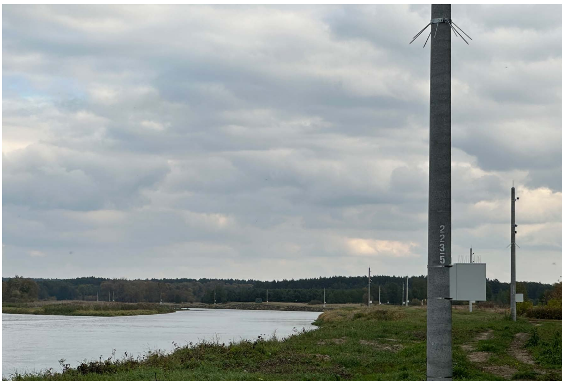
Figure 3.24. Photograph of the electronic barrier along the Bug River. Photograph by Peter Teunissen, March 2025.
